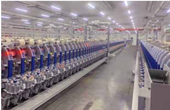
Project Name: Infinia Spining Mills Limited Financed By: Gulshan Branch, Dhaka & Jubilee Road Branch, Chattogram
